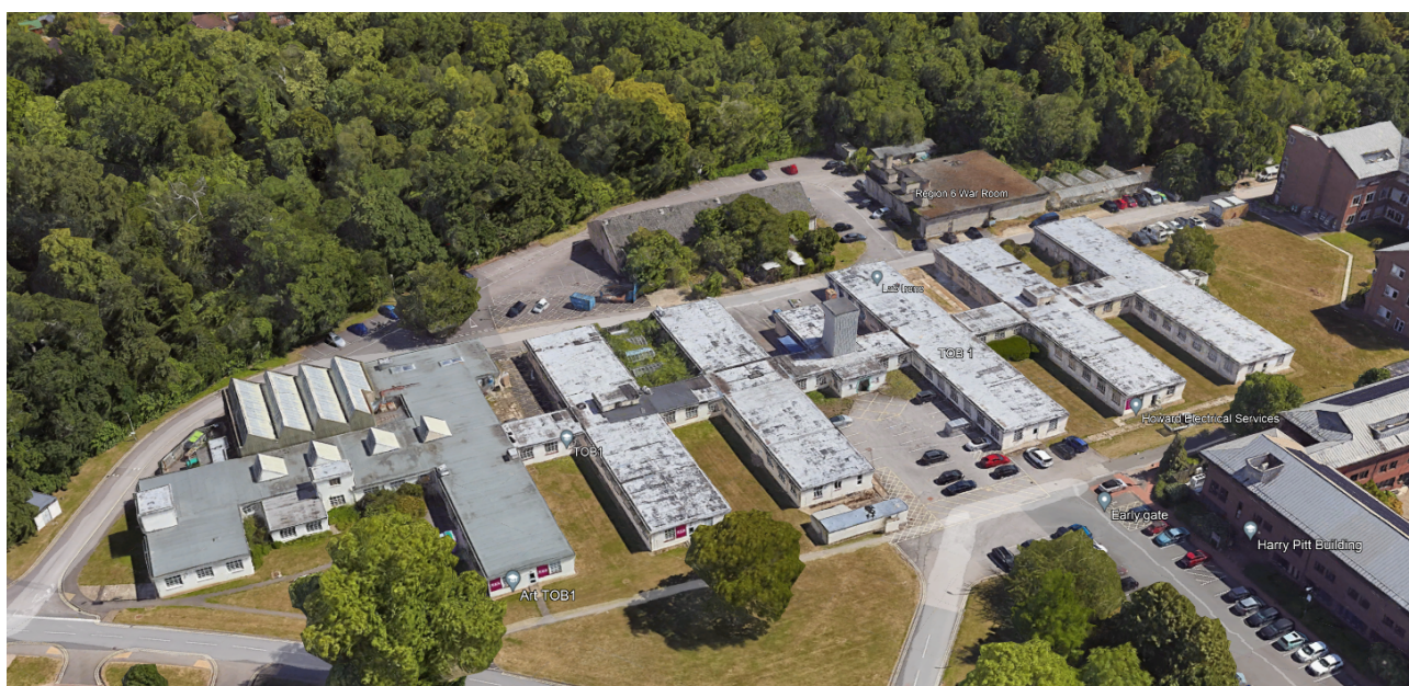
Figure 4: Temporary Office Building 1 to be demolished (TOB1)
