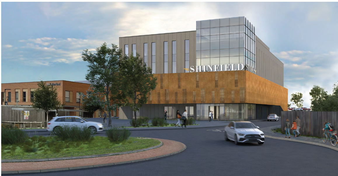
Figure 3: Proposed front elevation of the building taken from the internal Science Park roundabout. This shows the main glazed entrance and the ribbon of detailing above the first floor. The building sits well in the context of the Rutherford Building shown on the left.
