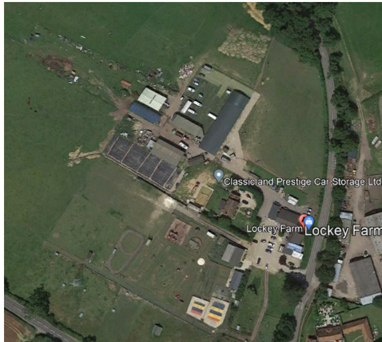
2022 aerial photo of the application site (Google Earth)
