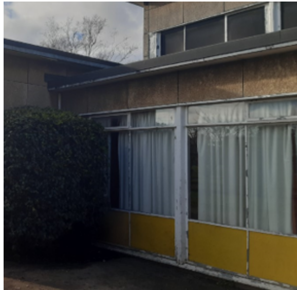
Photo 1: glazed windows to the west of the dining hall courtyard
