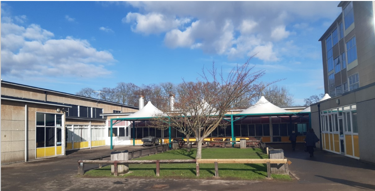
Southern coryard to rear of dining space with the original glazed screen across the low single storey dining element (and to range to LHS of image)
