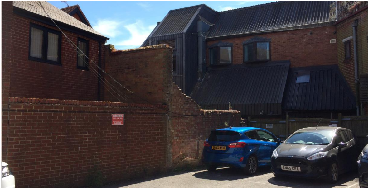
To 3-7 Easthampstead Road and the Ritz
