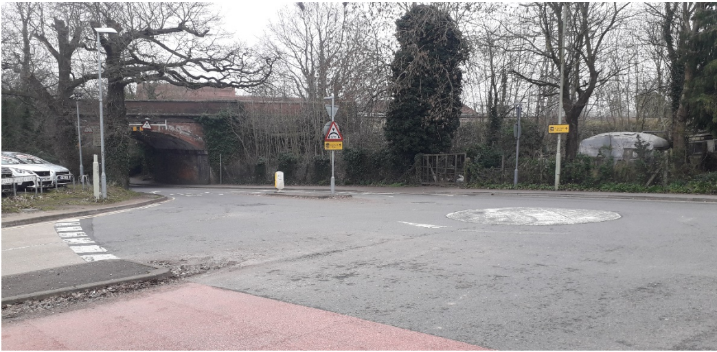
Mini-roundabout junction – from Molly Millars Lane, view towards Finchampstead Rd railway bridge
