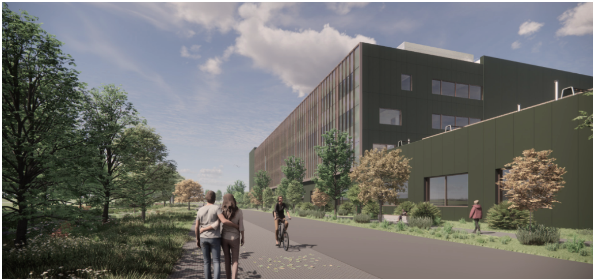
Figure 7: A perspective of the rear elevation of the facility
